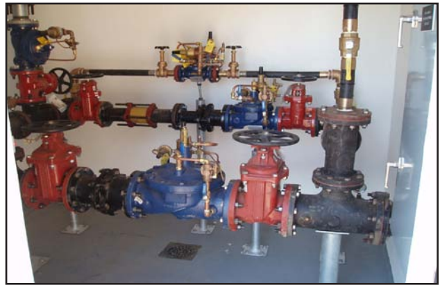
The view up at one of the new PRV vaults (left), and (top right) a look down toward Homer gives a sense of some of the challenges of the site. Multiple pressure-reducing valves (bottom right) are critical for the community's water delivery.
