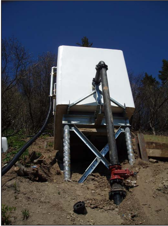
The view up at one of the new PRV vaults (left), and (top right) a look down toward Homer gives a sense of some of the challenges of the site. Multiple pressure-reducing valves (bottom right) are critical for the community's water delivery.
