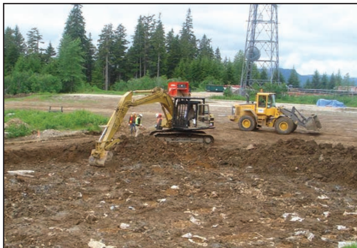
Site work continued in summer 2008.
