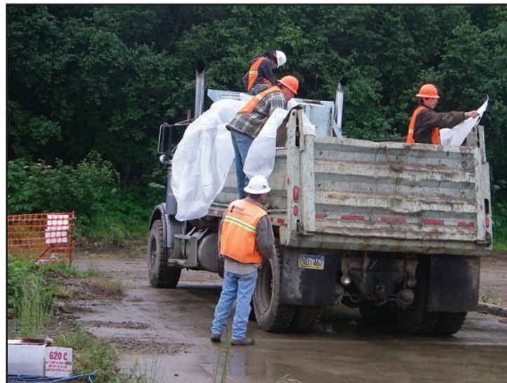
Bristol was responsible for determining logistics for excavation, transportation, and disposal of PCB-contaminated soil from this remote Alaska site.
